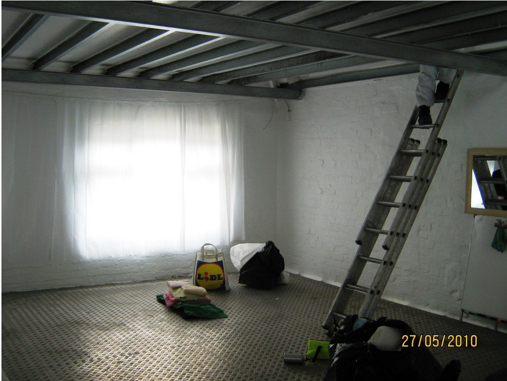
The front bedroom
